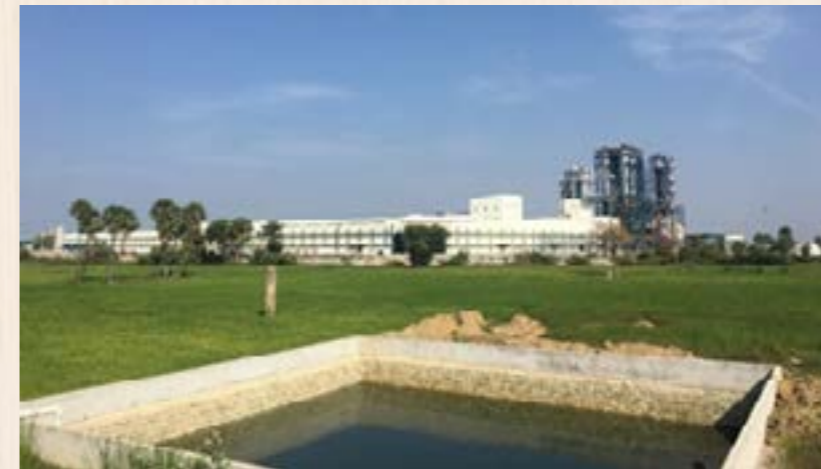
Constructed RWH pond
