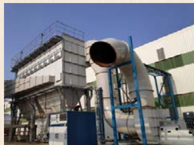
Installed bag house filter and present stack
